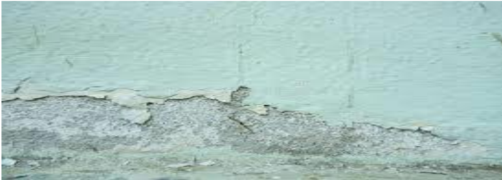
FIX PAINT DETERIORATION
